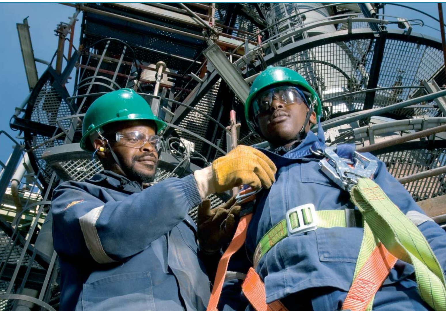
Two contractors checking a safety harness before performing maintenance activities during a planned shutdown at the Sasol Solvents plant in Secunda.
