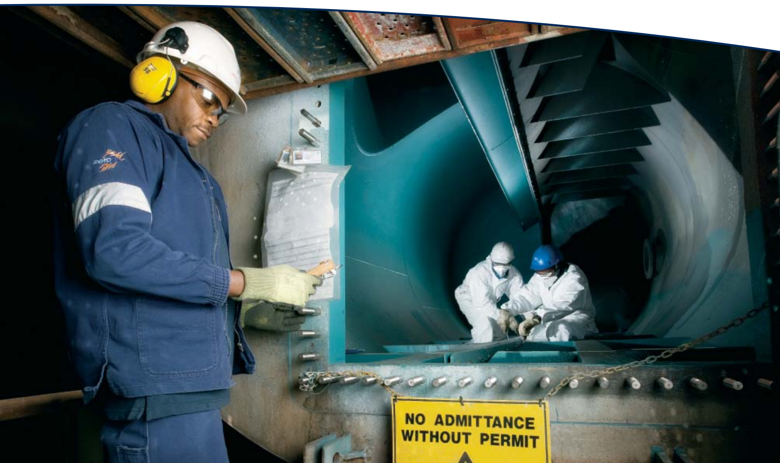
Lucas Mngomezulu, production standby, checking for the possible presence of gases in a vessel that requires special safety measures for confined space entry.
